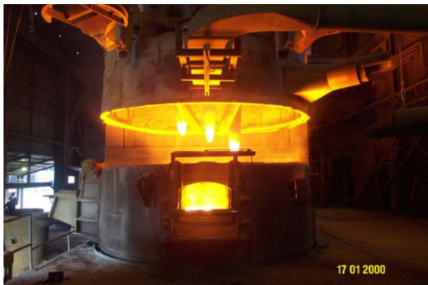
1 Electric arc furnace for refined ferromanganese production
